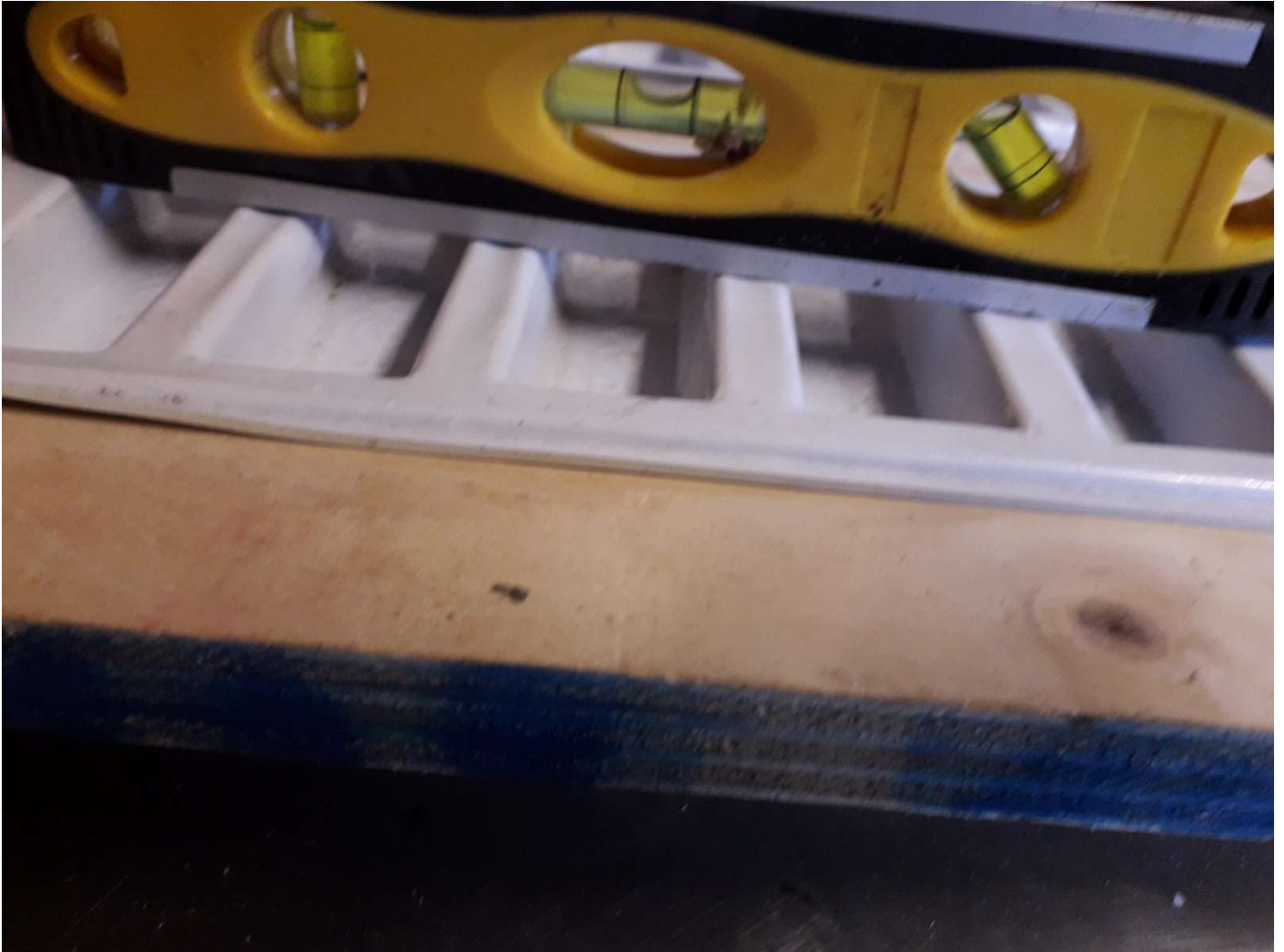
Use a spirit level to ensure eve moulding. Photo: John Goodwin.
